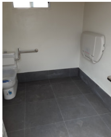
"Toilet block interior for Recreation Facility."
